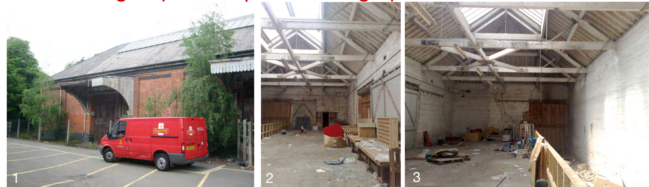
Photographs of the existing 1879 Railway Goods Shed Grade II Listed
